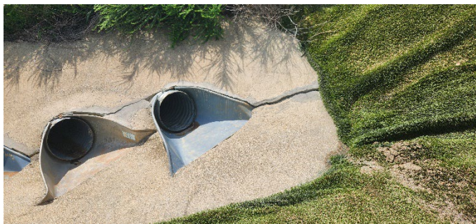
Headwall Cracks
