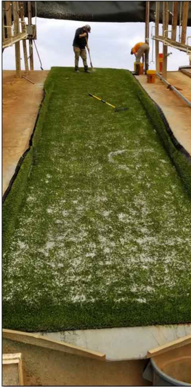
(a) Infill Installation
