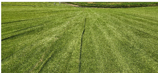
Turf Wrinkles in Landfill Slope
