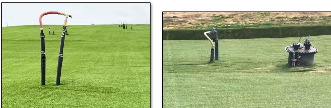
Figure 7-2. ClosureTurf Integrated with Landfill Gas Collection System
